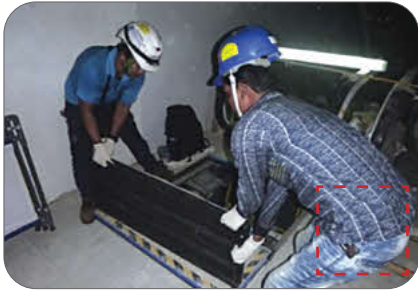
Figure 22: Risk of back injury when lifting heavy load.
