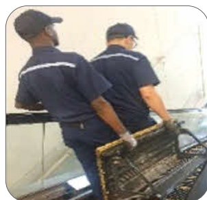
Figure 21: Risk of foot injury when load drops.
