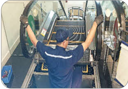
Figure 11: Fall when getting in/out of escalator machine room/pit.
