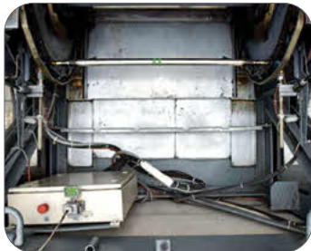
Figure 32: Good housekeeping for the pit.
