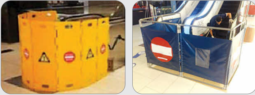
Figure 26: Barricade to prevent unauthorised entry.
