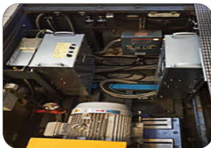
Figure 18: Knocking on equipment parts and tripping on trunking due to lack of space in the escalator machine room.
