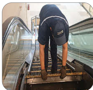
Figure 19: Risk of back injury when lifting heavy load.
