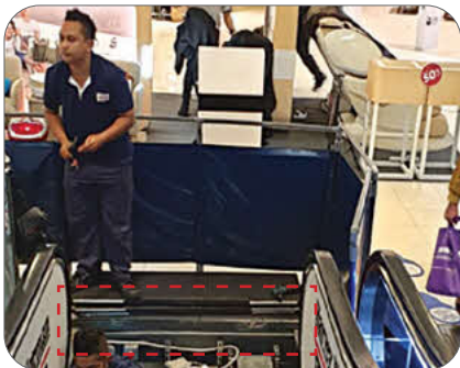
Figure 24: Limited working area beyond escalator pit.
