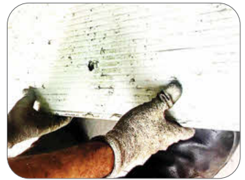
Figure 28: Wear hand gloves when handling floor plates.
