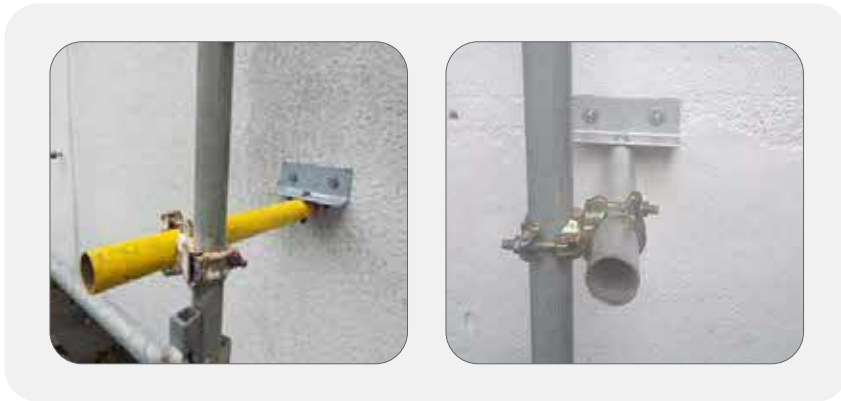
Figure 3: Examples of additional tie-backs for scaffolds
