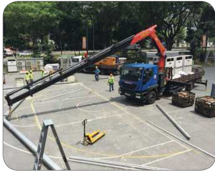
Figure 9: Lorry crane lifting tent frame members.
