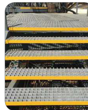
Figure 8: Warning strips on steps.
