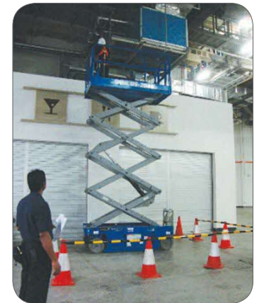
Figure 12: Work zone cordoned off.
