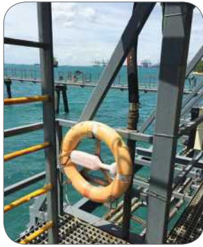
Figure 30: Edge protection and buoy.
