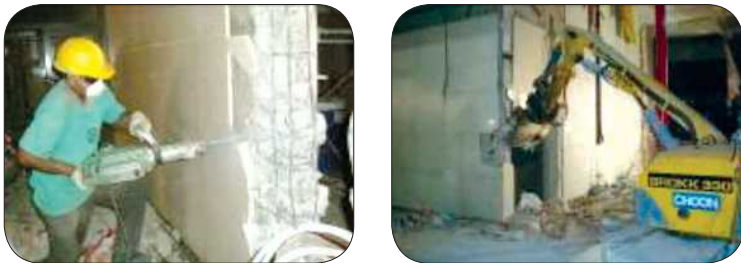
Figure 2: Substitution of jack hammer (left) with automated machine (right) to break concrete reduced the noise level from 90 dB(A) to 83 dB(A).
