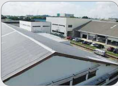
Wide-spanning metal roof of industrial building.
