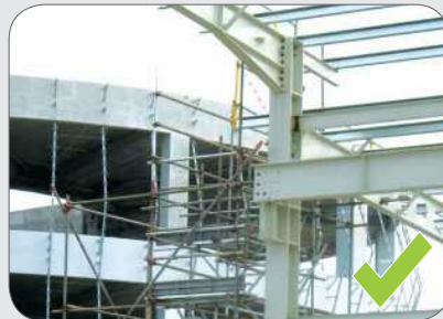
A properly constructed scaffold with hand holds and guardrails for safe access to the roof.
