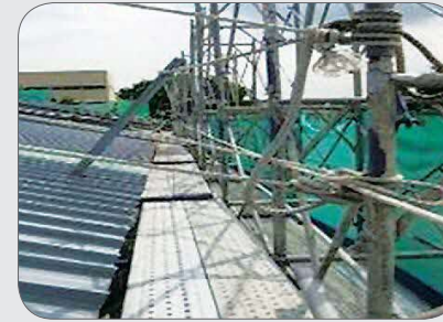
Scaffolds offering roof edge fall protection.
