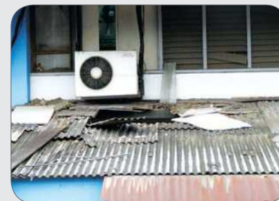
Old corrugated roof sheets.
