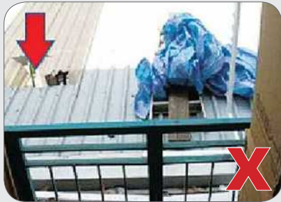
Fragile roof surface is not identified before work and no safety signage is used to warn workers of hazard.
