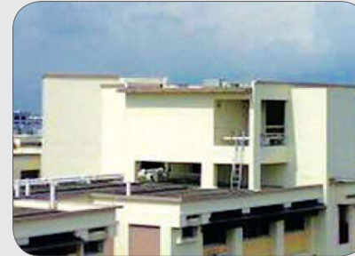
Flat non-fragile roof with low parapet walls.
