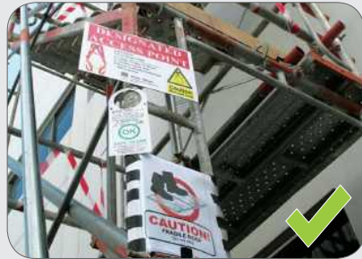
Fragile roof surfaces are identified and warning signage is provided at designated access point(s) onto roof.
