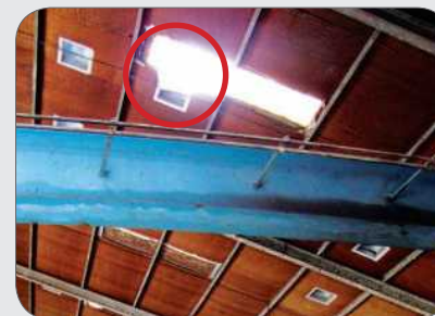
Example of skylight on factory roof.
