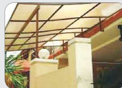
Car porch with polycarbonate roofing.
