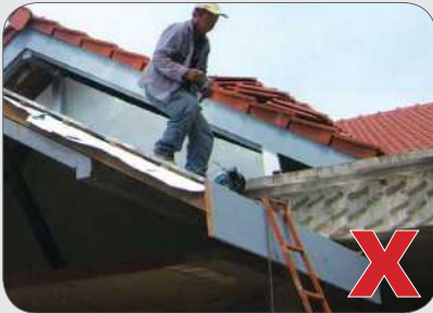
Roof access ladder is not secured to structure at bottom and top rungs.
