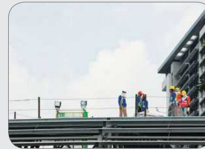
Guardrails erected on roof surface.
