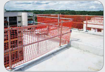
Guardrails erected at edge of flat roof.
