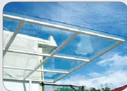
Glass canopy roof of car porch.
