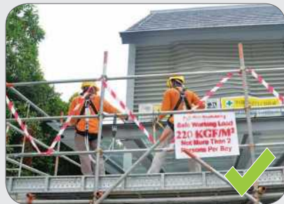
Installation of glass canopy roof with proper access and work platforms.
