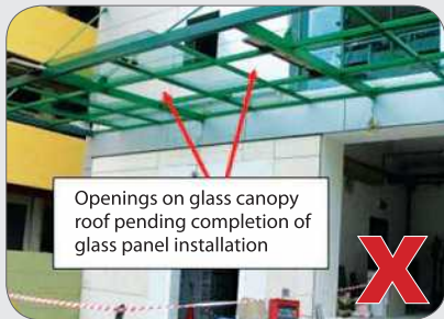
Installation of glass canopy roof without proper access and measures against falling through roof openings.
