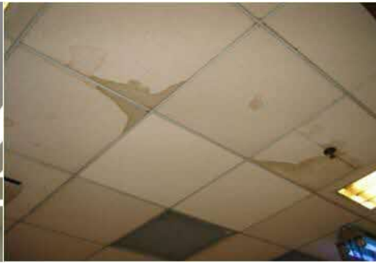
Figure 5: Water marks on ceiling board may indicate leakage from water pipe.
