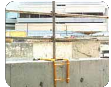
Figure 31: Example of parapet edge protection design.
