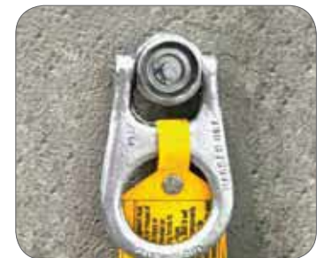
Figure 2: Example of a cast-in eyebolt anchor.
