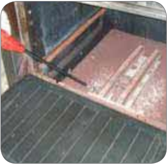
Figure 30: Lighting of pilot flame using a handheld spark generator
