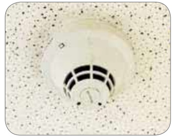
Figure 12: Ceiling-mounted smoke detector
