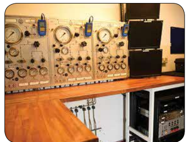
Figure 5: Dive control panel with monitor and communication recording system.
