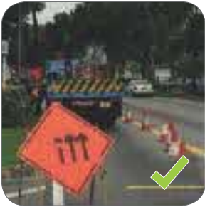
Figure 111: Warning signs help alert oncoming traffic.
