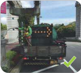
Figure 17: Place warning signs at prominent locations and directional arrows to alert and divert traffic.
