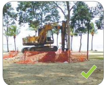
Figure 55: Barricade work area with warning tapes and signs.
