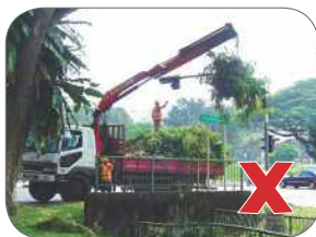
Figure 50: Do not stand below suspended load or on top of unsecured load at all times.
