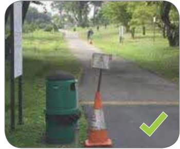
Figure 27: Place warning signs to re-direct the pedestrian.
