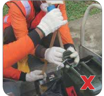
Figure 86: Incorrect gloves used for handling petrol.
