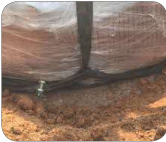
Figure 60: Suitable capacity slings coupled together with rated load; suitably rated webbing straps should be added by attaching to lower slings at base of root ball, lacing and tightening over top of root ball to prevent lower slings at base, from slipping beneath the load. Refer to Figure 63.
