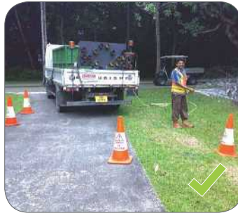
Figure 18: Cordon off work when carrying out stationary watering.
