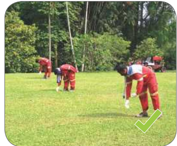
Figure 20: Inspect the turf area for foreign items such as rocks and nails prior to starting work.
