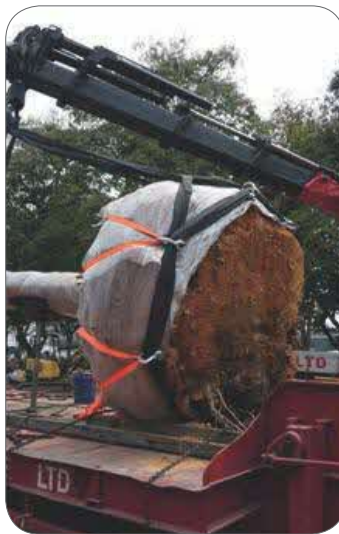
Figure 63: Illustrates lacing from over top of root ball (orange webbing) to prevent lower slings at base, from slipping beneath the load.
