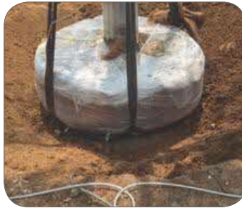
Figure 61: Vertical lift slings arranged evenly around the root ball to form the cradle or basket to be lifted.
