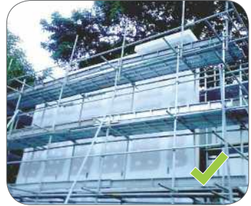
Figure 15: Install guard rails and toe-boards on scaffolds.
