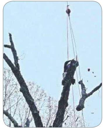
Figure 44: A crane is used to lower the cut portion.
