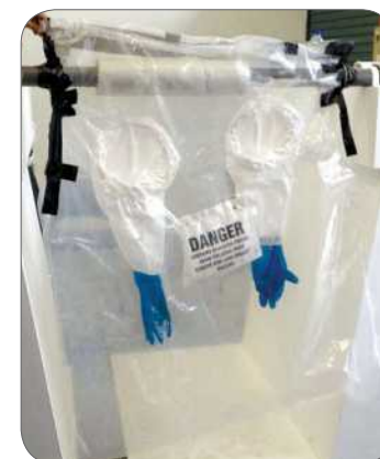
Figure 15: Glove bag containing asbestos waste.
