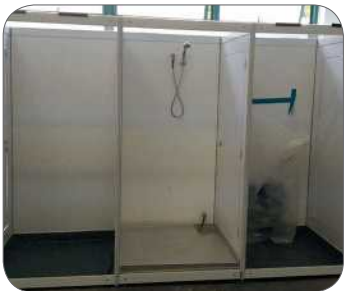
Figure 13: A decontamination facility consisting of three separate compartments (clean, shower and dirty areas).
