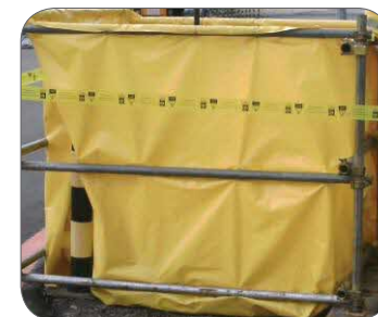
Figure 9: Example of a self-supporting temporary enclosure.
