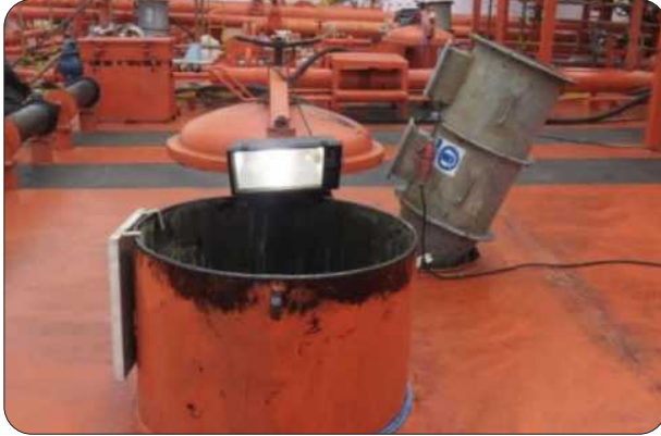
Figure 14: Access point into the tank.
