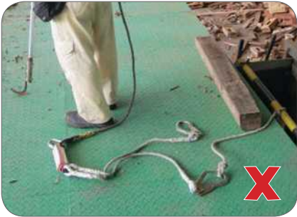
Figure 41: Example of an unsafe practice showing extension of a travel restraint length with incorrect usage of a twin lanyards system.
