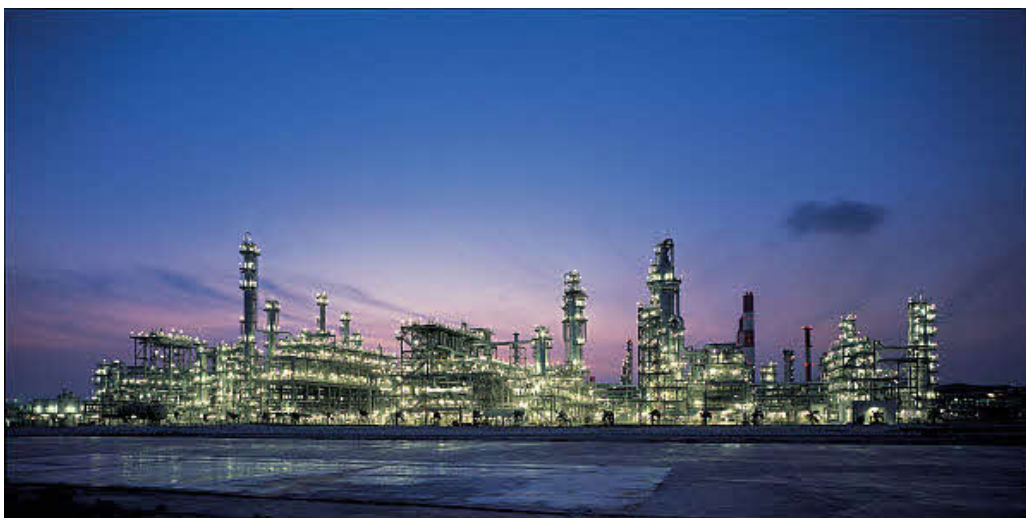
Figure 1: A typical oil refinery
