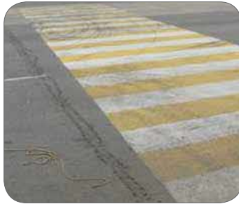
Example of a demarcated walkway.
