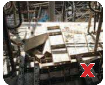
Figure 17: Unsecured materials placed near edges may be knocked over accidentally.
