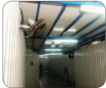
Figure 15: Collective protection is achieved by use of an adequately robust overhead shelter.
