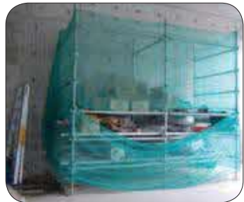
Figure 7: Netting can help prevent the dislodging of stored items.
