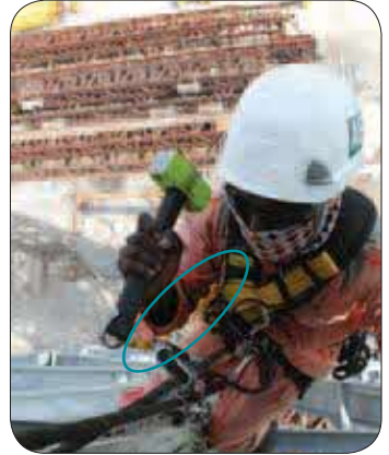
Figure 11: Tools tethered to the user by means of a lanyard can prevent them from falling and striking persons below. It also prevents them from being left behind accidentally after work.
