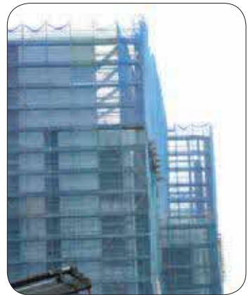
Figure 8: Overlay nets can prevent light objects from being accidentally thrown from the interior of the building.
