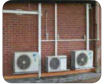
Figure 3: Air-conditioning compressor units installed at ground level eliminates the need for work at height and the risk of being struck by falling objects.
