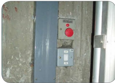
Figure 96: Emergency stop & lighting button switch with easy access
