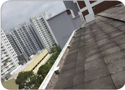
Figure 28: Falling off from open sides at the roof or from edges of buildings
