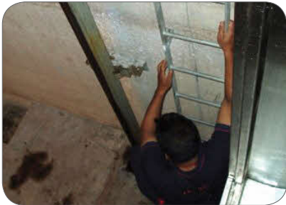
Figure 93: Pit ladder in good condition
