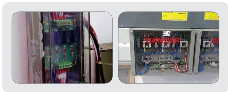
Figure 73: Examples of clear labelling, finger safe terminal block (plastic covering)
