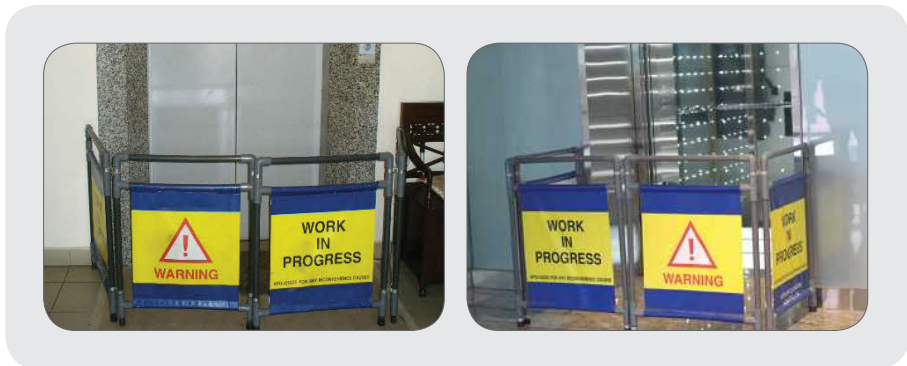
Figure 86: An example of using lift barrier to warn the public of falling hazards at lift landings
