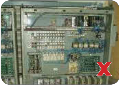
Figure 19: Electrical panels without covers can expose workers to electrical hazards
