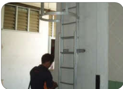
Figure 56: An example of cat ladder with guard & proper handhold
