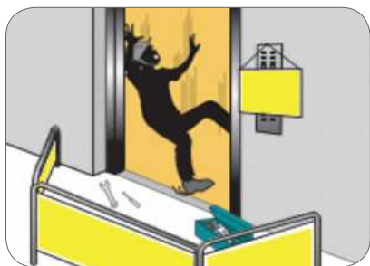
Figure 34: Falling through the open landing door into the hoist way
