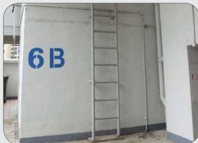
Figure 41: Examples of vertical cat ladder (without safety cage) to access to lift motor room on roof top may be dangerous with risk of falling
