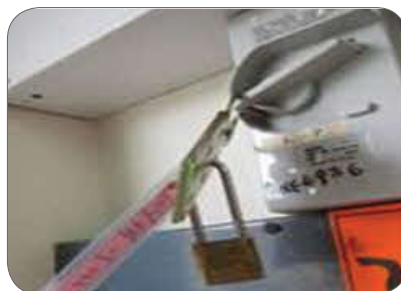
Figure 106: Example of lockout-and-tagout
