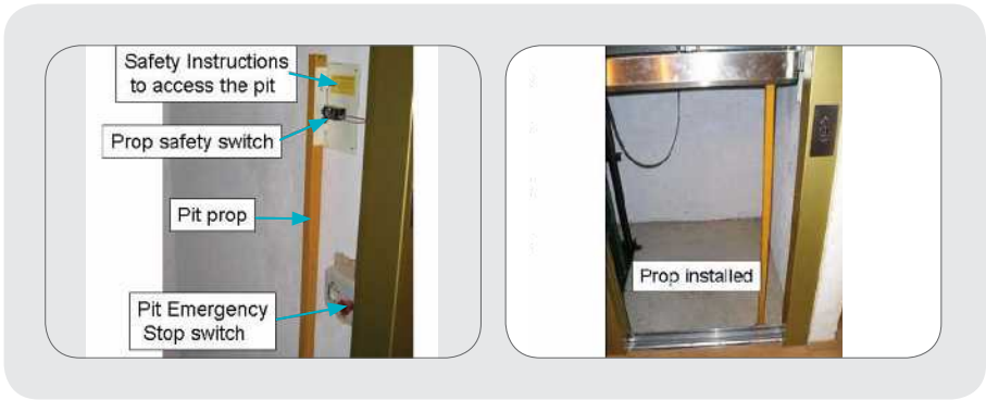
Figure 92: Prop along the wall or guide rail for home lift
