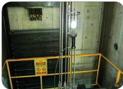
Figure 83: Car top brightly lit with LED lighting, visible signage, and barricaded
