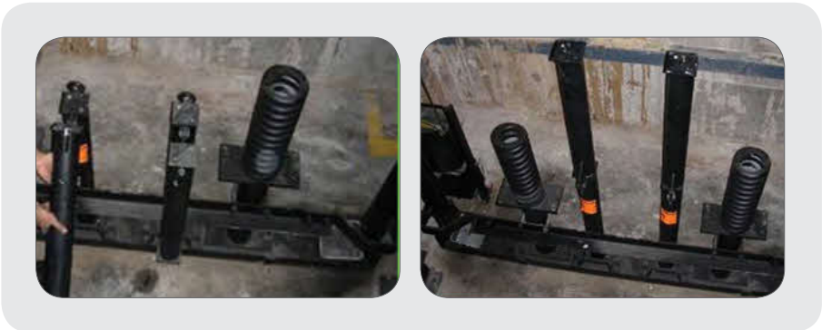
Figure 91: Pit props located in pit under the car in the middle of the pit for hydraulic lift
