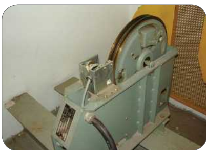
Figure 16: Fingers may get pinched at the moving parts that are left uncovered
