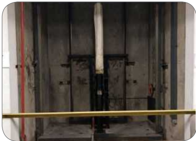
Figure 88: Door access to lift pit more than 2.5 metres
