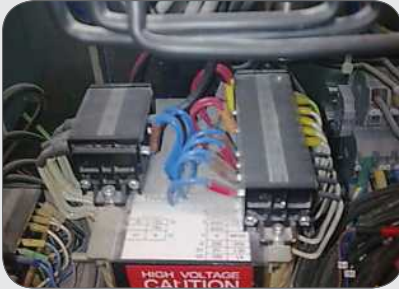
Figure 76: Examples of clear marking and labelling on electrical wires and terminations
