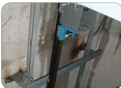
Figure 27: Worker can get electrocuted when he comes into contact with a damp hoist way
