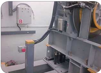
Figure 69: An example of an emergency stop switch next to the drive sheave
