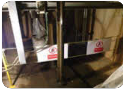
Figure 90: Safety fencing in lift pit at multiple lift shafts
