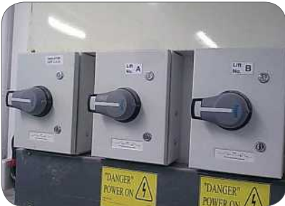
Figure 77: Examples of clear marking on lift isolators and distribution boards
