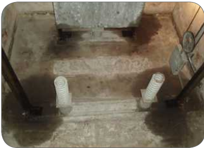
Figure 95: Clean & well lighted pit
