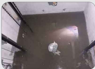
Figure 25: Flooded lift pit
