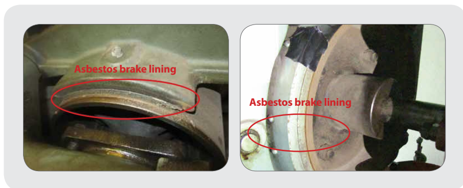
Figure 50: Examples of asbestos brake lining found in lift motors
