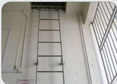
Figure 41: Examples of vertical cat ladder (without safety cage) to access to lift motor room on roof top may be dangerous with risk of falling
