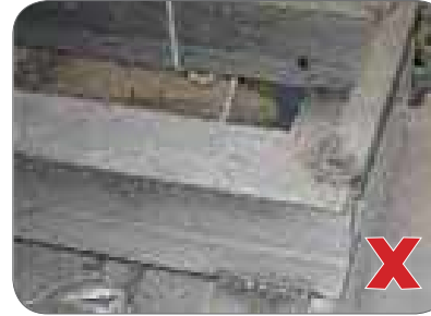
Sharp corners (cutting hazards).
