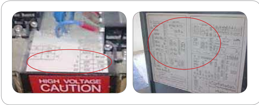
Figure 51: Examples of clear marking and labelling on electrical wires and terminal blocks.
