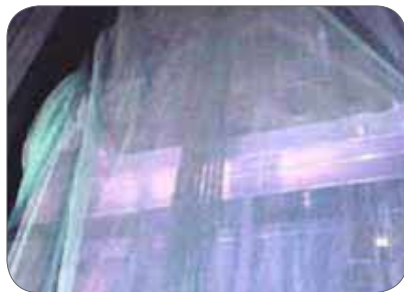
Figure 37: Netting partition used to isolate hoist way to prevent workers from being hit by items accidentally dropped from other hoistways.
