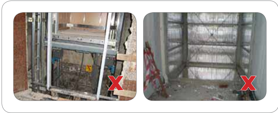
Figure 22: Falling into the hoist way from lift landings.
