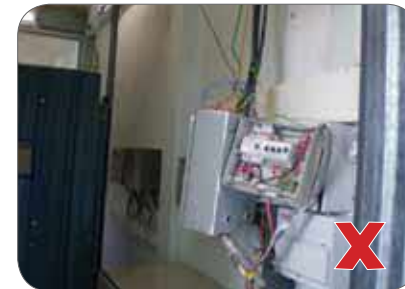
Figure 17: Worker can get electrocuted when he comes into contact with defective electrical equipment.
