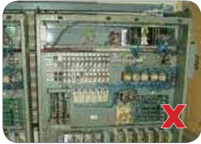
Figure 10: Electrical panels without covers can expose workers to electrical hazards.
