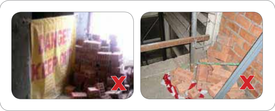
Figure 33: Equipment or materials falling through landing door into hoist way.
