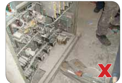
Figure 18: Worker can get electrocuted when he comes into contact with exposed electrical terminations.
