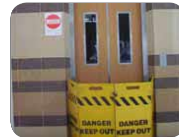
Figure 57: An example of using lift barrier to prevent unauthorised access.
