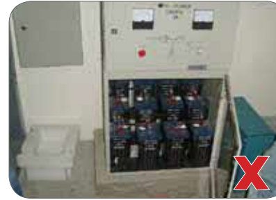
Figure 16: Electrocuted when worker comes into contact with improper insulated emergency battery operated power supply (EBOPS).
