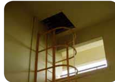
Figure 47: Example of cat ladder with ringed hoops.
