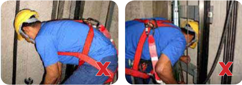
Figure 34: Hit by stationary bracket when the lift moves.
