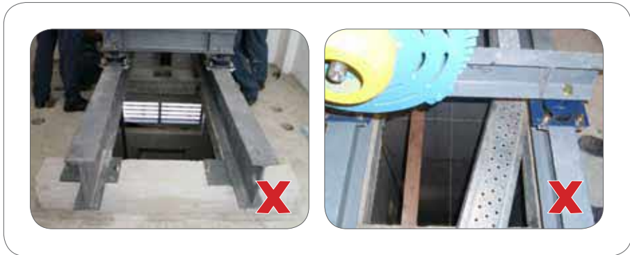
Figure 25: Falling through openings in machine room floor that were not properly covered during lift installation work.
