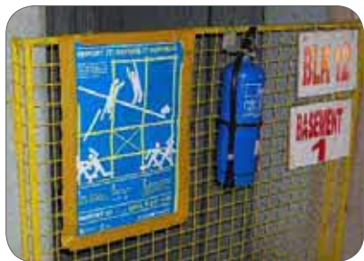
Figure 55: Example of shaft entrance protection.
