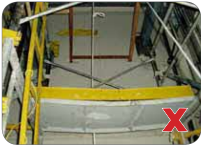
Figure 24: Falling off improperly constructed platforms and ladders when worker is using them to help replace ropes, sheaves, and so on.
