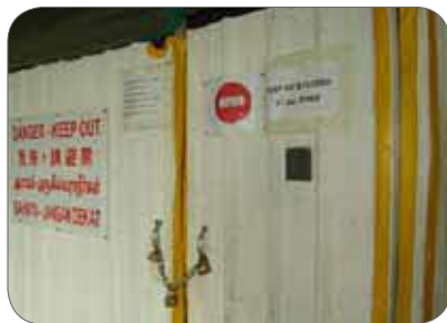
Figure 56: Example of hoarding during lift modernisation.
