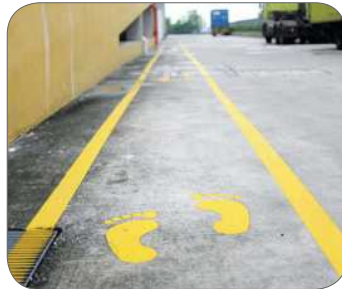
Figure 11: Demarcated pedestrian walkway.
