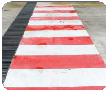
Figure 12: Demarcated pedestrian crossing.
